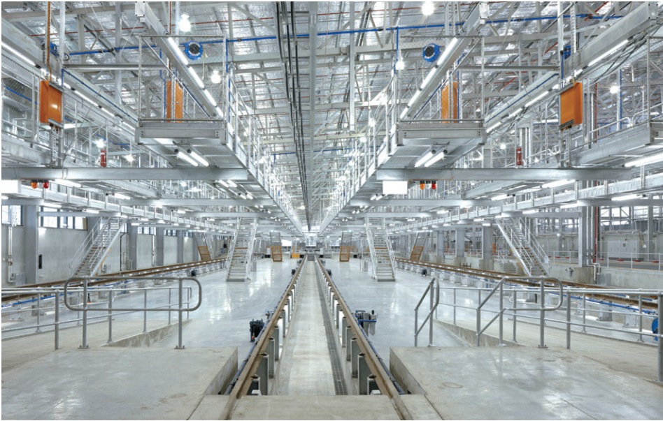
Inside of Craigieburn Train Maintenance Facility.
